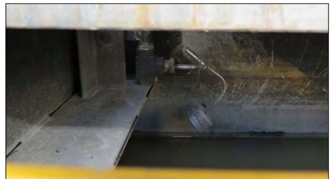
Typical Automatic Float Switch In Sump
