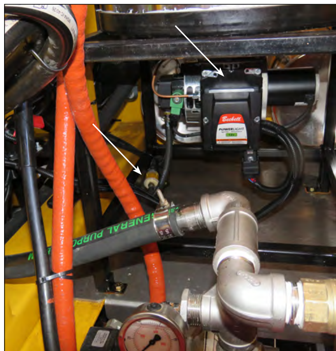
Water Heater Fuel Oil Burner & Fuel Filter
