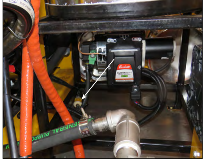
Water Heater Burner & Burner Fuel Filter
