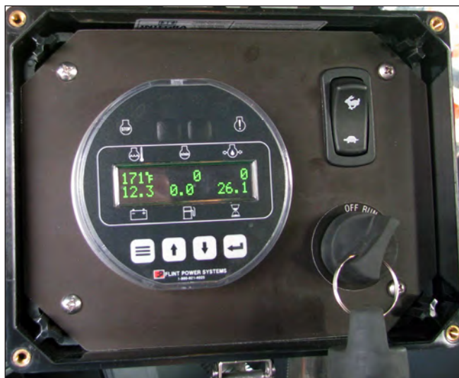
Auxiliary Engine Control Panel & Ignition Key Switch
