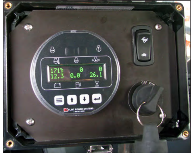
Auxiliary Engine Control Panel
