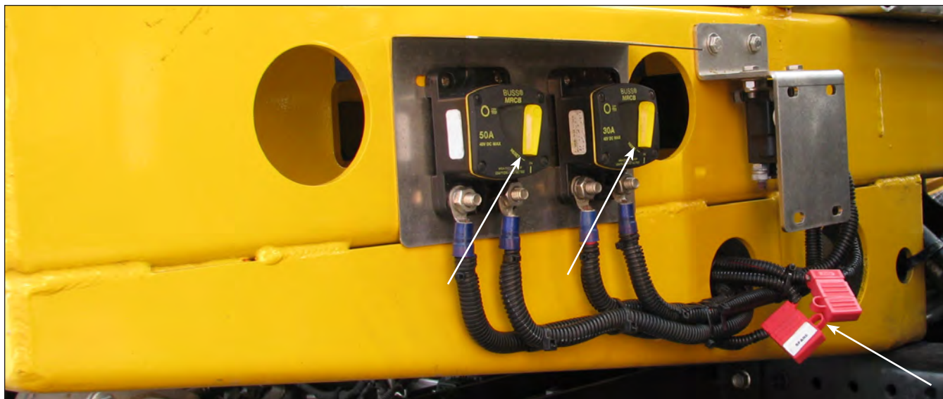
Main Circuit Breakers & In-Line Fuses
