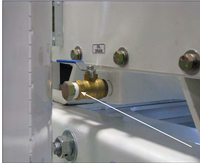
Crankcase Oil Drain Valve & Safety Plug
