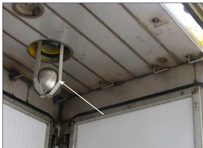
Stainless Steel Vacuum Cutoff Ball Valve
