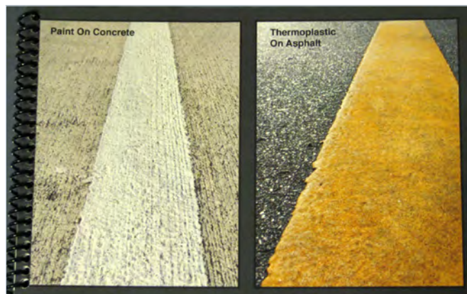
Paint On Concrete /Thermoplastic On Asphalt
