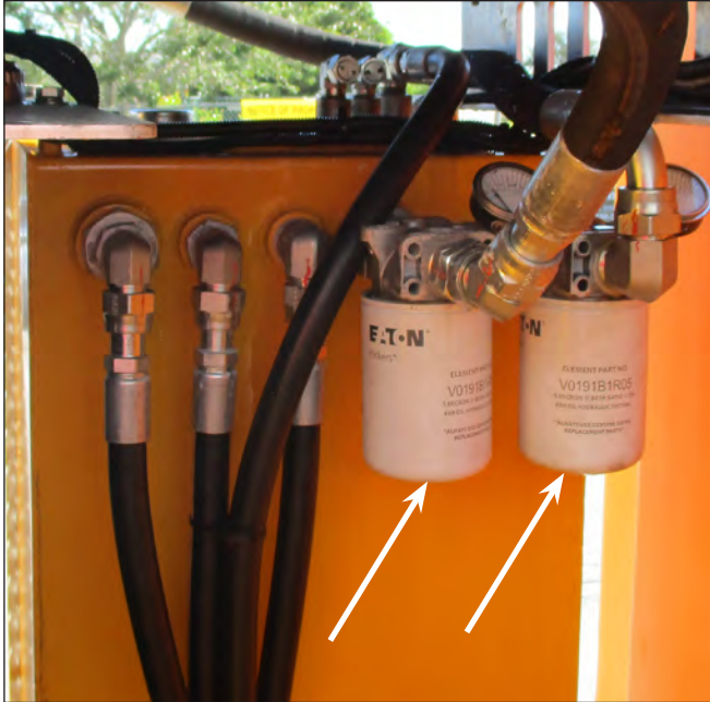
Low Pressure Return Filters & Gauges On Hydraulic Reservoir
