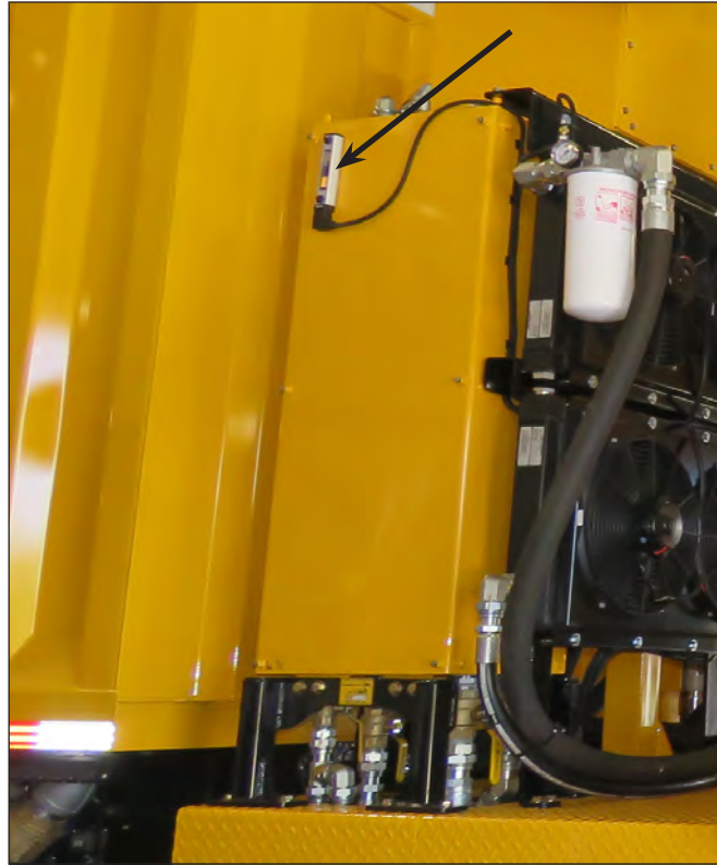
Hydraulic Fluid Reservoir & Sight Glass
