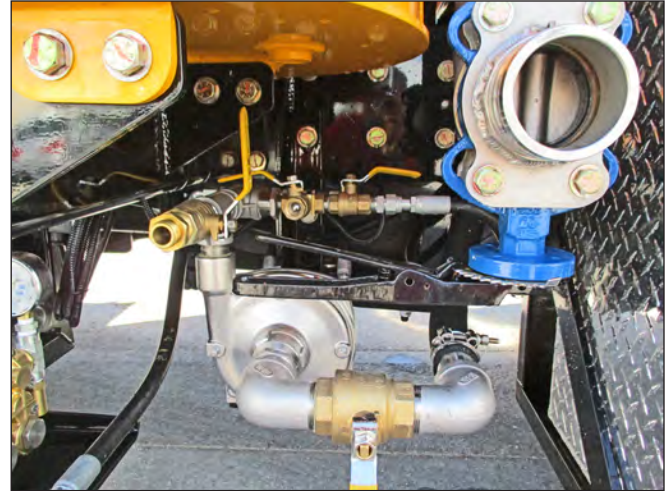
Water Pump Washdown Hose Connection
