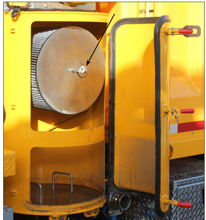
Service Port Plug Installed
