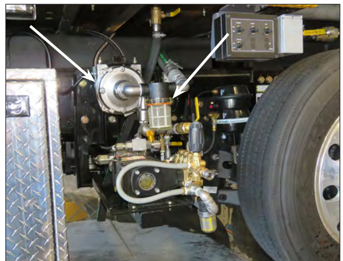
Water Pump & Water Strainer
