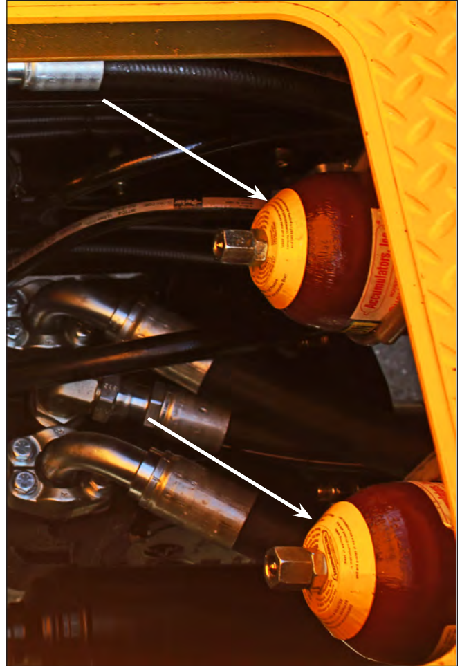
Cutter & Skip Cylinder Accumulators Below Access Plate In Center Deck
