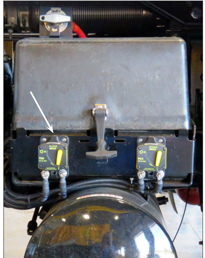
Main Circuit Breakers
