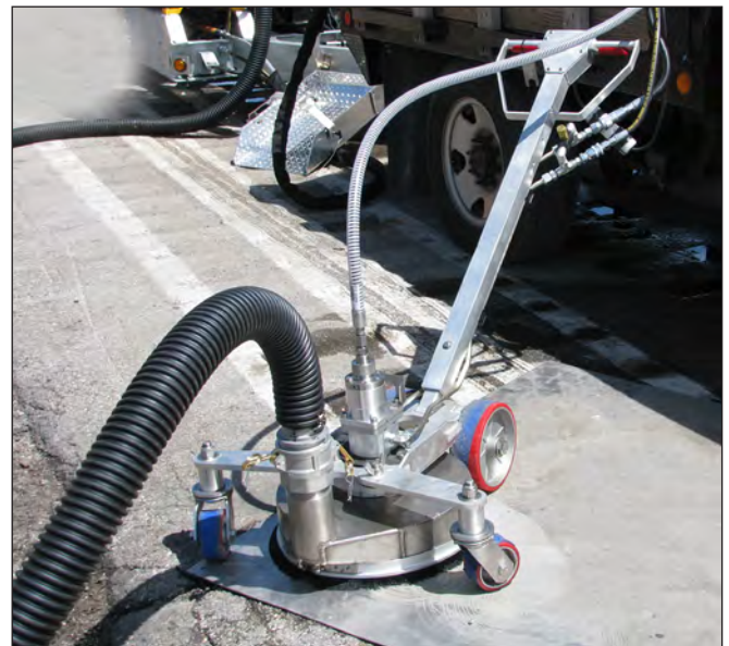
Ground Hog With Hydraulic, Vacuum & UHP Hoses Connected
